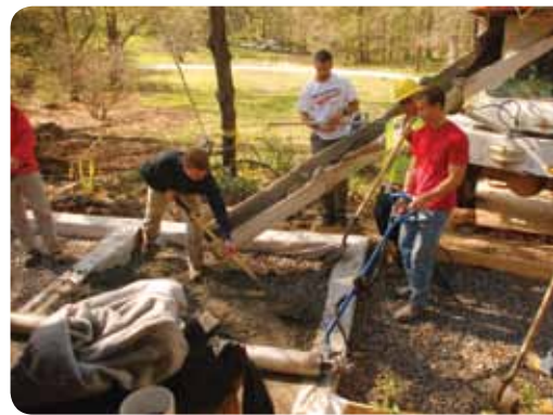
Michael Hein's Reinforced Concrete Structures students work on pouring pervious concrete for the walkway that passes in front of the Arboretum Pavilion.
