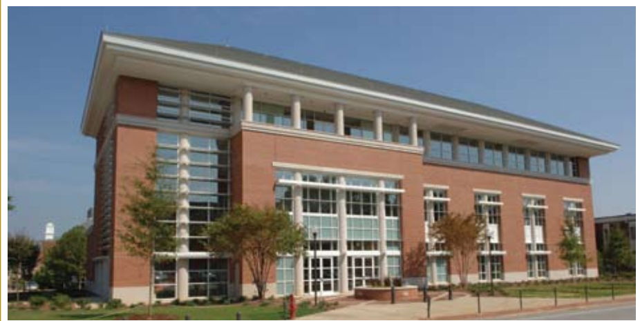
With rapid progress over the summer, exterior work has been completed on the Miller Gorrie Center, the new home for the Department of Building Science in the College of Architecture, Design and Construction. Advanced technologies taught in the college were used in construction of the $9.3 million facility, which is set for completion in October.
