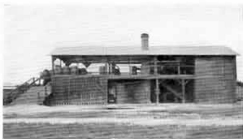
Fig. 15. This modern plant, near Gainesville, Florida, has one of the government style still settings and approved Bureau type shed, which takes the lowest possible insurance rate. Approximately 90 government style still settings have been built but this shed represents recent modern developments. Note the protective tin roof over the wing walls.
