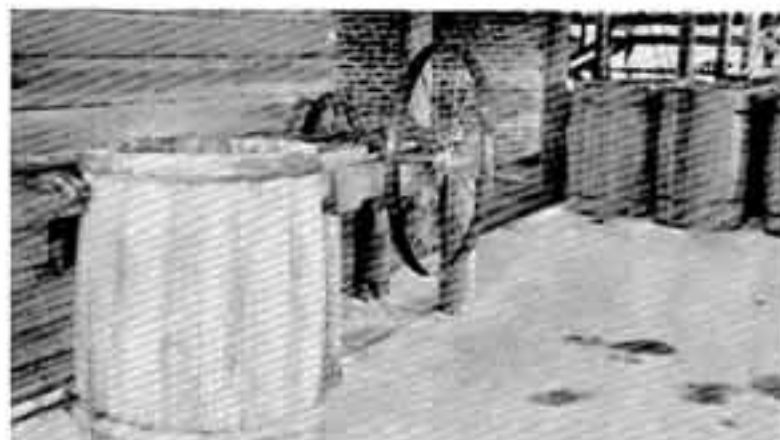
Fig. 18. Cooper's winch made from salvaged gears gives the cooper ten times the power that the old wheel provided. Durable tight barrels can be made with this set-up. Space under the main still shed is utilized for this cooper shop.
