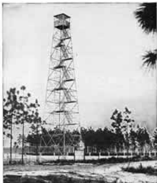
Fig. 13. "THE EYES OF THE SERVICE." During the fire season, lookouts man the 50 observation towers and locate fires when they are small. Telephone connections to organized crews aid the Florida Forest Service and landowners in suppressing the fires before much damage is done.
